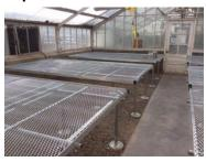
The Structural Maintenance shop performed the installation of new benches in the Fabian Garcia Horticulture Farm building 158 Greenhouse. This project required assembling the benches and pouring the mounting piers. This was performed in all four rooms of the greenhouse. The team was recognized by Dr. Geno Picchioni, Plant and Environmental Science Professor, for a job well done and appreciation for their dedication to providing a quality product.
